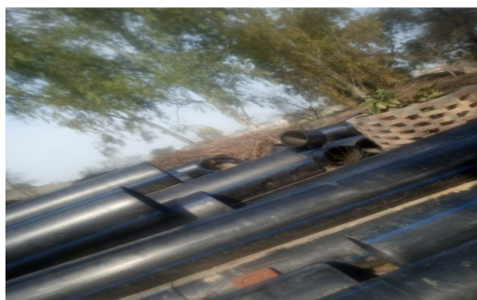
Pipes lying in Nangla village
